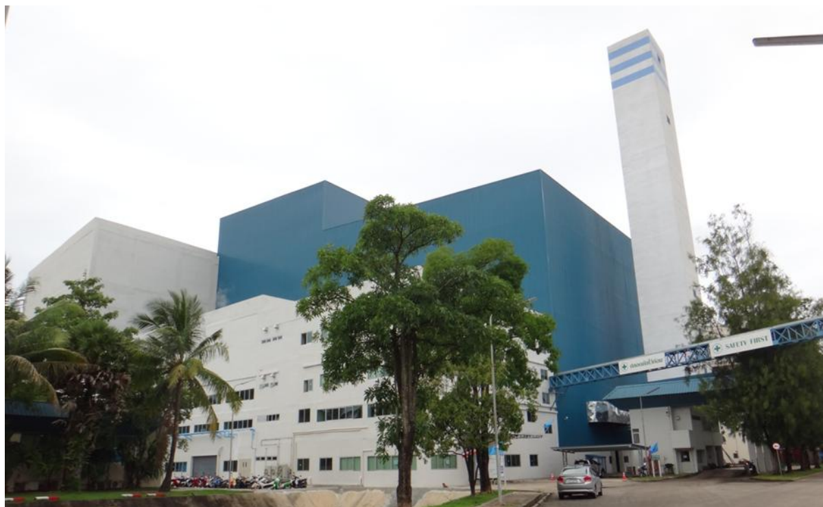
PHUKET MUNICIPAL SOLID WASTE INCINERATION POWER PLANT
